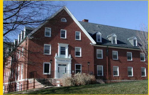
Dorchester Hall Renovation (2018)
