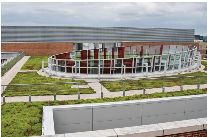
Rainwater Harvesting (Example: Physical Sciences Complex Green Roof)
