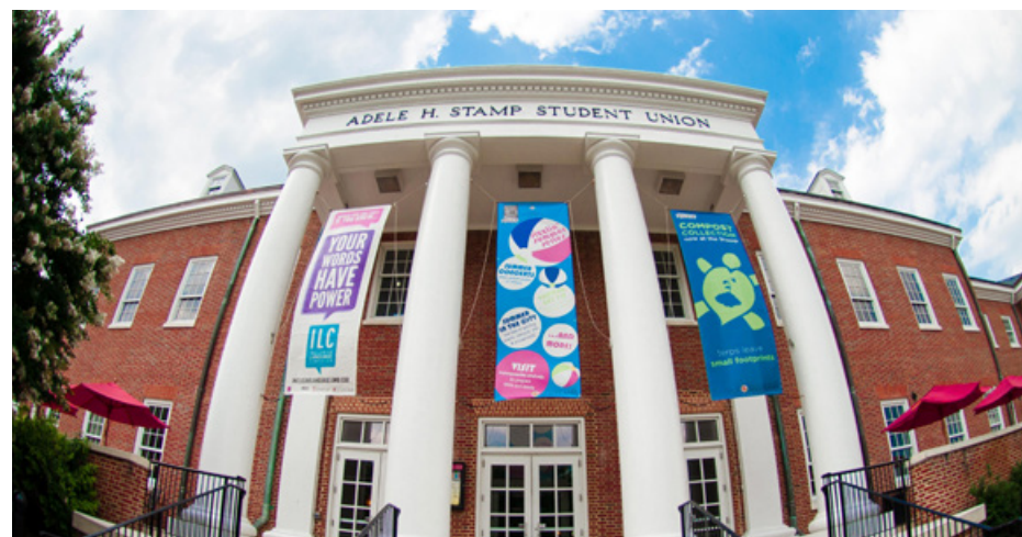
A new transit plaza at Stamp Union will further-strengthen its presence as a key hub of activity for UMD
