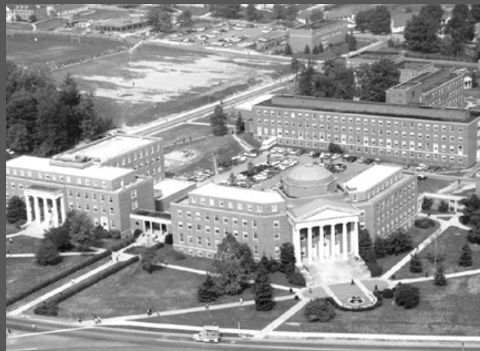
Martin Hall (1950) and Kirwan Hall (1954) with interior parking courtyard, reflecting transition to car-oriented development.
