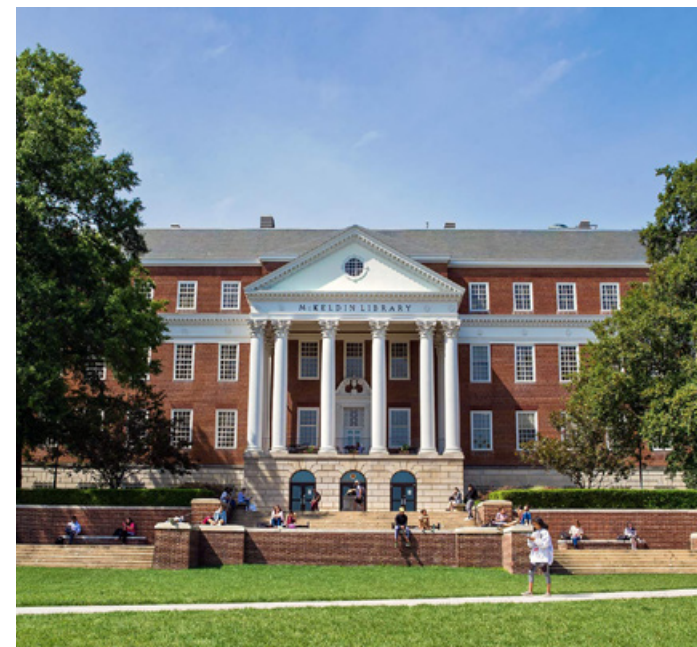
McKeldin Library currently has an FQI rating of 73-100, and is also considered an “iconic” campus building
