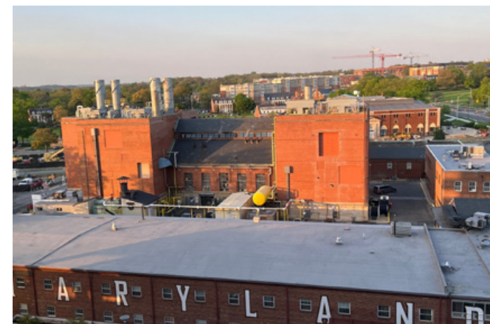
The Energy Plant, or CHP, produces steam and electricity from natural gas
