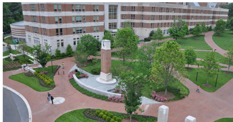
The extension of Mayer Mall will further strengthen the identity of the South Campus Village
