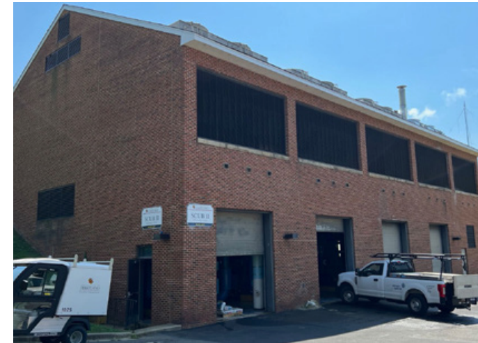
SCUB II: 32 Year-Old Facility Serving Within the Campus Core
