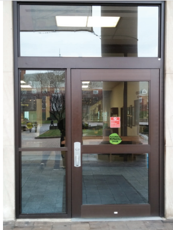
Entrance Type: Secondary Mid-Century Modern / Contemporary Hornbake Library 147
